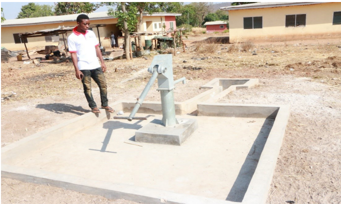
The completed hand-pumped borehole at Jama Newtown
