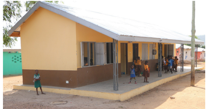
Renovated Kindergarten block at Jama Newtown
