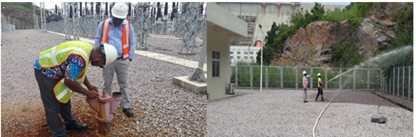
Inspection and testing of Fire Hydrants
