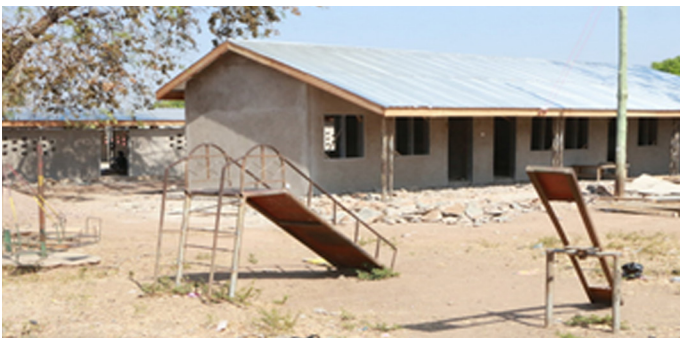
Renovation works on the Kindergarten at Jama Newtown
