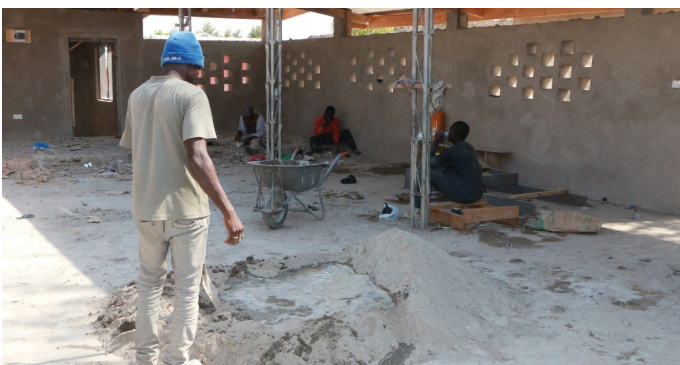
Renovation works on the Community Centre
