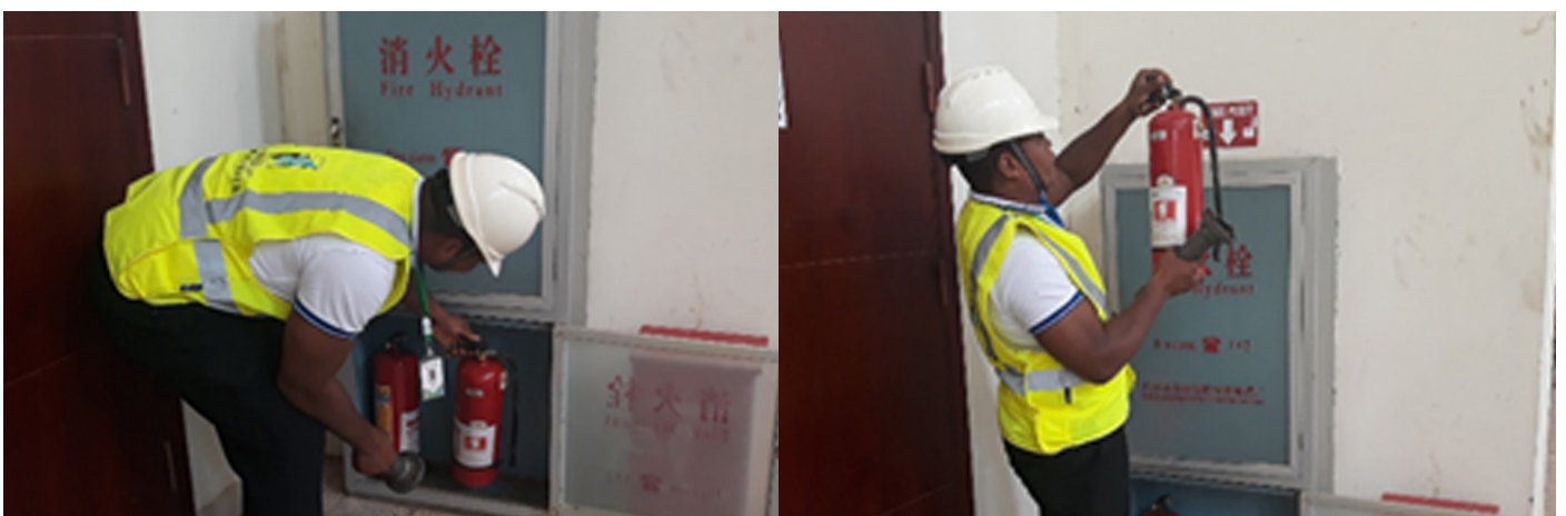
Routine Inspection of Firefighting Agents
