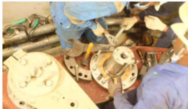
Figure 15: Installation of new stem housing
