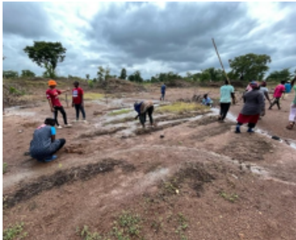
Figure 44: Contractors undertaking line and pegging on the field
