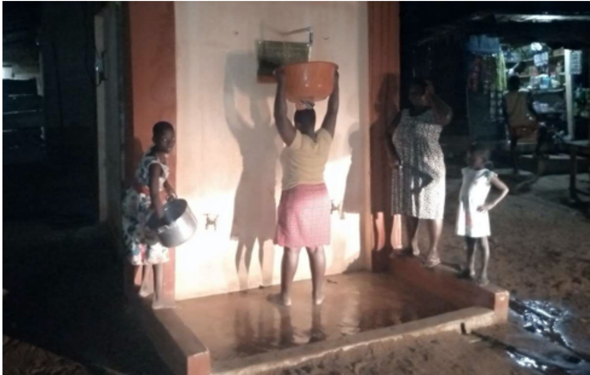
Figure 32: Mechanized borehole in use
