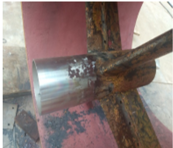
Figure 23: Stainless steel pipe (welded)
