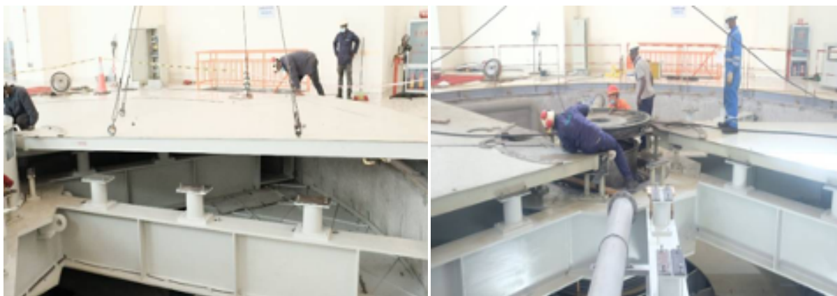
Figure 16: Setting of run-out test
