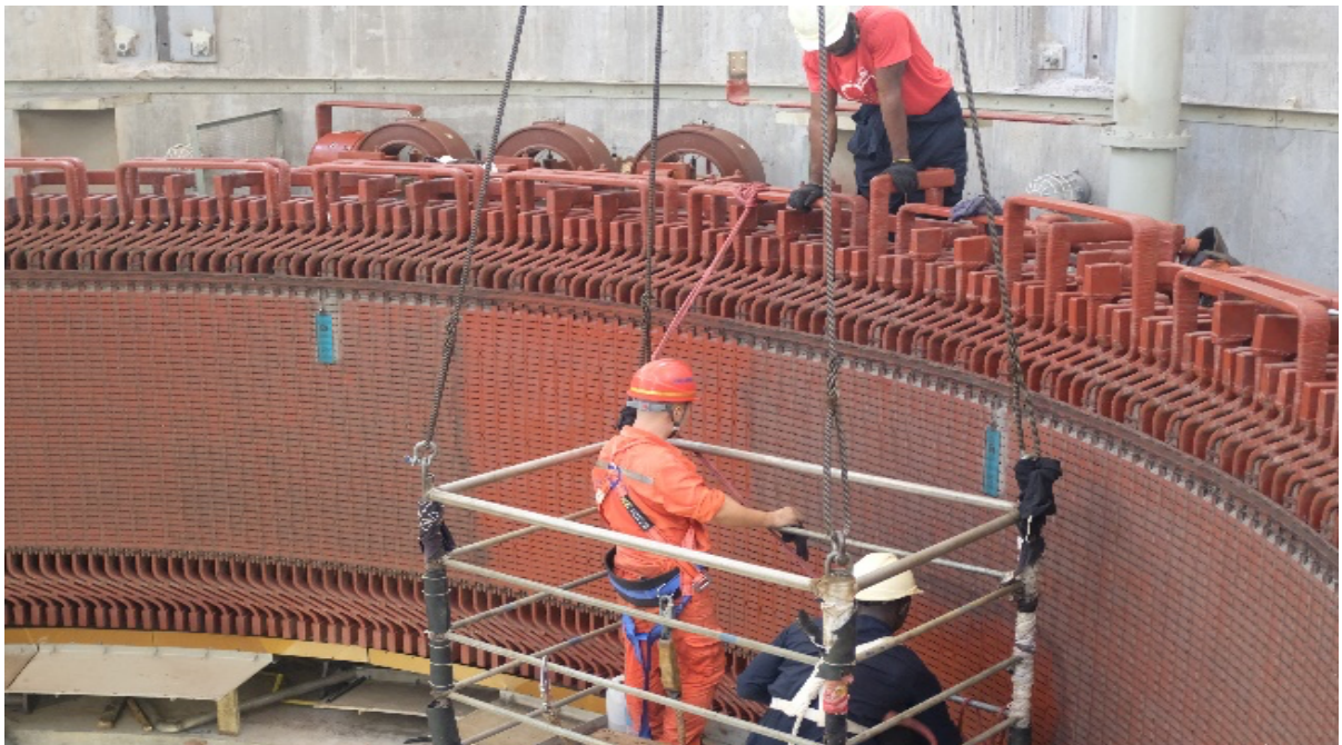
Figure 11: Visual Inspection and Cleaning of Generator Stator
