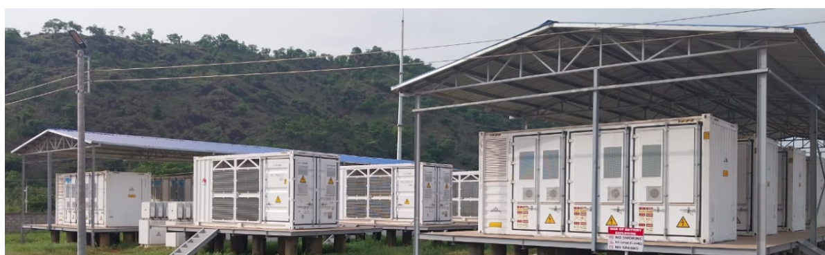
Figure 20: Battery storage for solar operations
