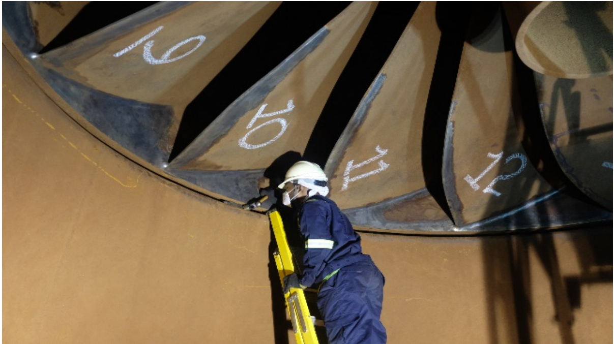
Figure 10: Polishing of the Turbine Runner Blades.
