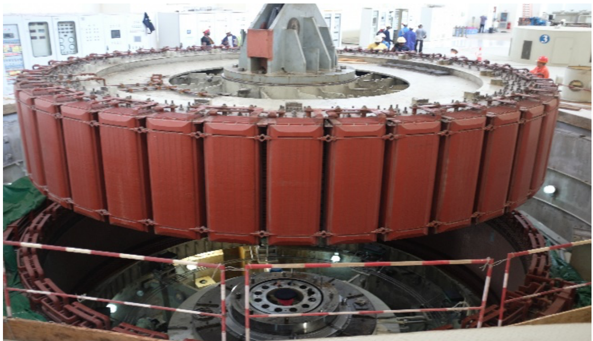
Figure 9: Lifting of the Generator Rotor from the Unit Assembly
