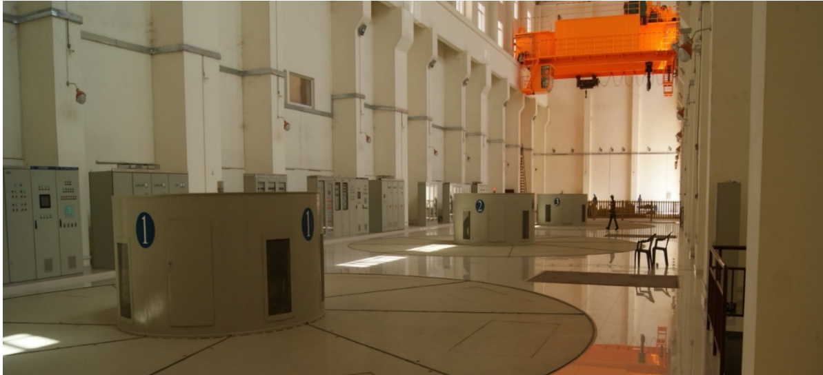
Figure 7: The BGS generator floor showing the three main hydro generating Units (i.e., Unit 1, Unit 2 and Unit 3)
